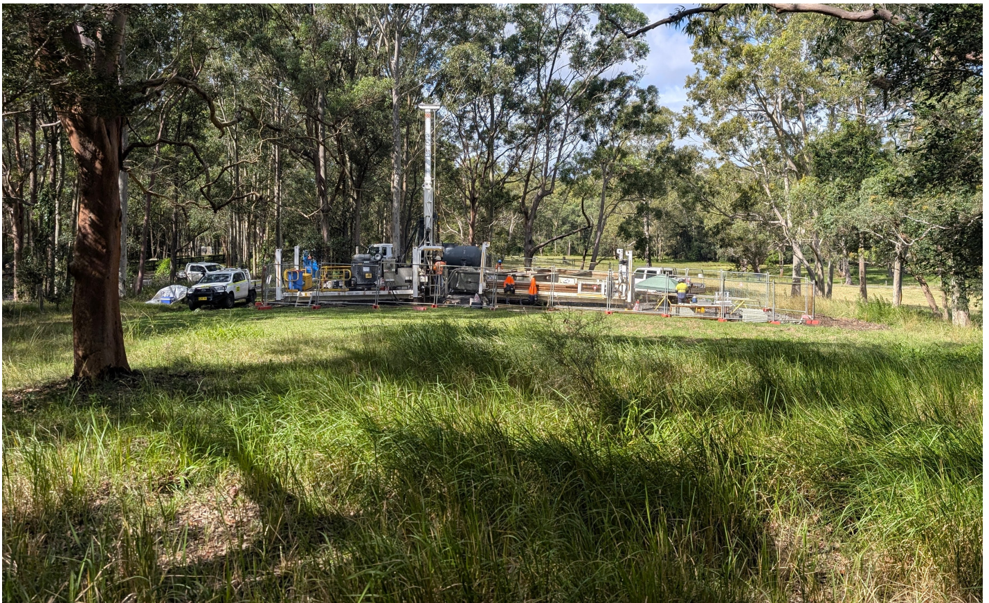
Typical layout of a exploration drill rig (Mandalong 2025).
